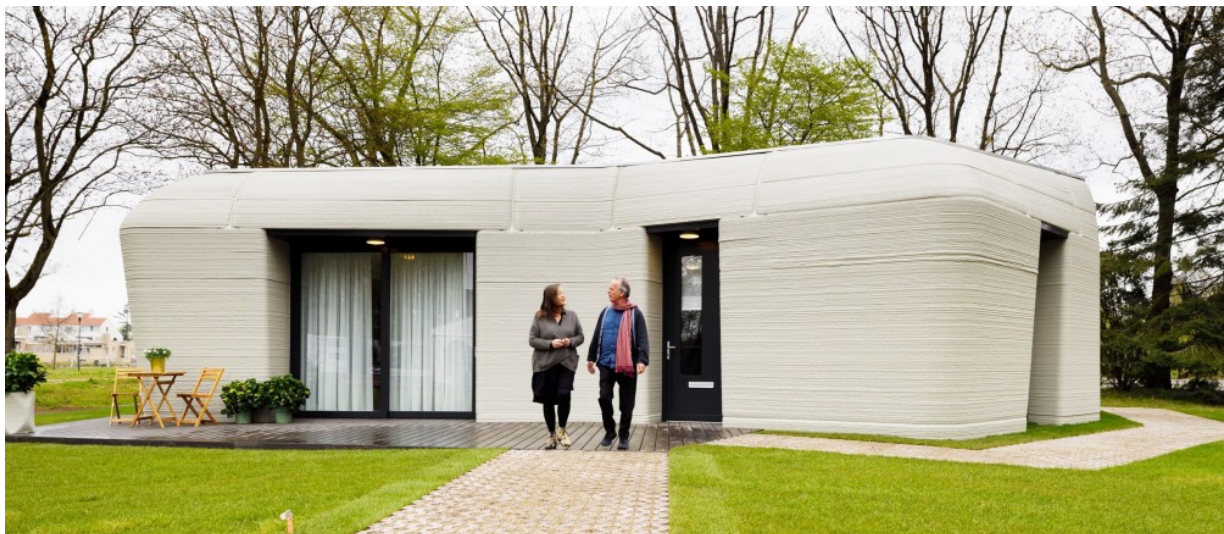
Abbildung 9: Project Milestone: First commercial 3D printed concrete house Quelle: 3D Printed House NL
